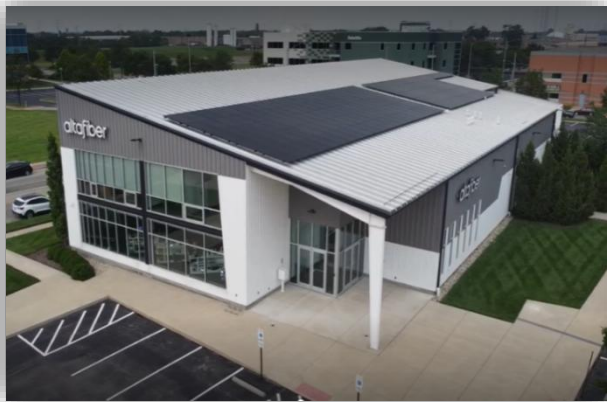
Figure 16: A 70.5-kW solar PV array powers the LEED Silver certified Dayton office and store. It is a net zero building.
